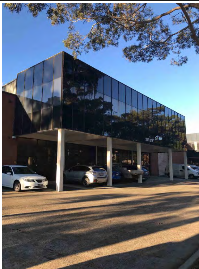
Photo 1: Facing south east onto north west area of building.
