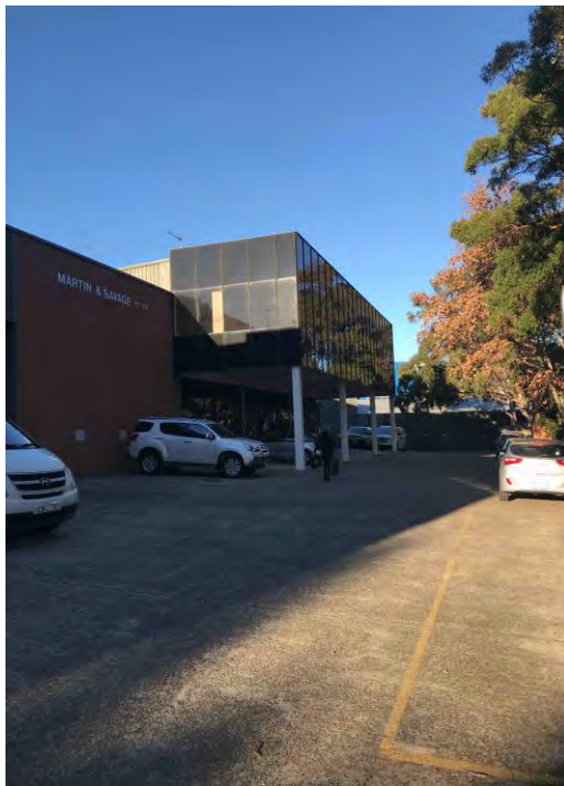
Photo 5: Car park in north west area of the site.
